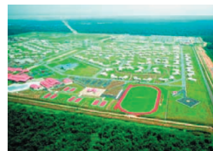
Bonny Island residential facilities
